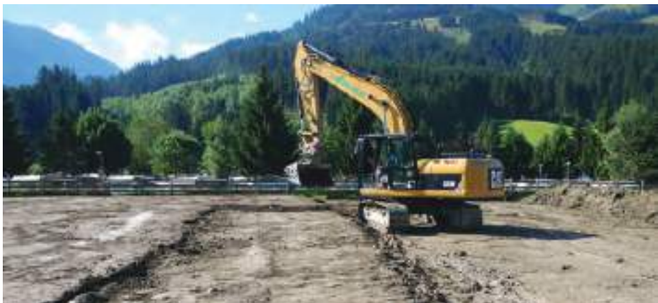
Figure 29: A positive example of soil treatment: The loosening of compacted soil followed by filling of underground and top soil in layers (Photo: Thomas Peham).
