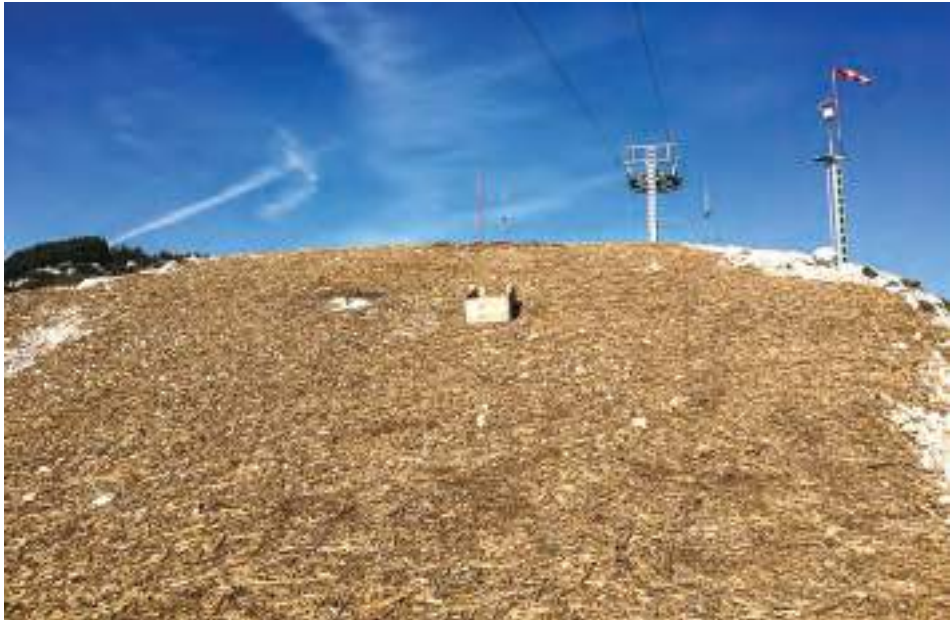
Figure 57 : Covering a ski slope that is almost without soil with wood-chips – an initial activity towards gradual restoration of grass cover; Vogel ski area.
